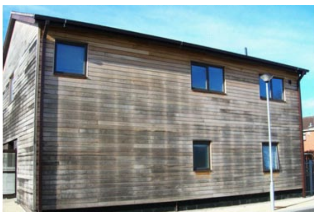
Figure 4 Light vertical lines on close-jointed oak cladding
