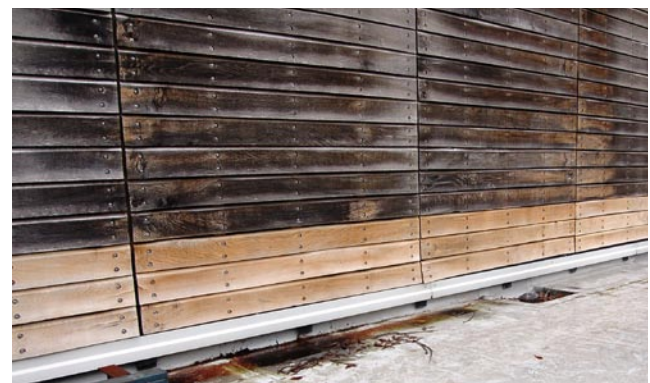
Figure 10 Test bays on oak cladding immediately following cleaning and treatment
